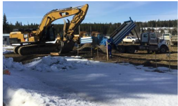
Heavy equipment inspected to ensure they are free of leaks.
