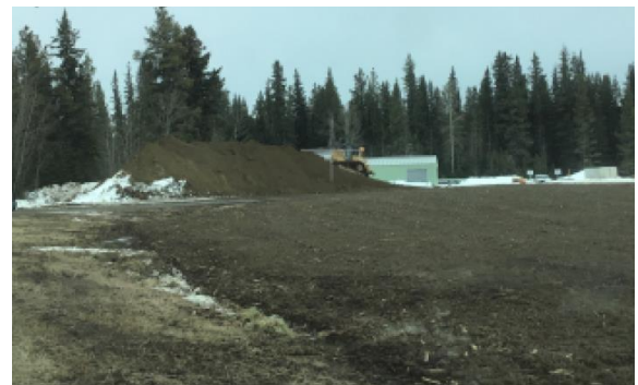
Topsoil and transition soil salvage piles, site graded.
