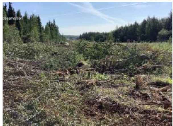
Brushing activities on the right-of-way.
