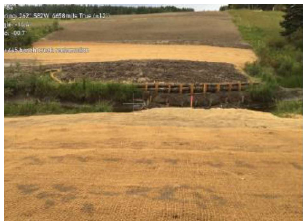
Creek fortification nearly complete and to be monitored during construction.
