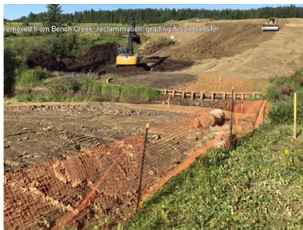
Backfill and grading activities on the right-of-way.
