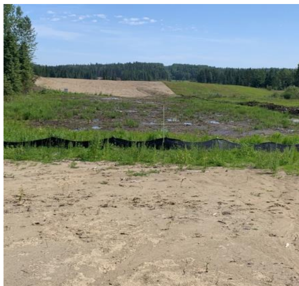
Wetland identified on-site with sediment control measures and good housekeeping.
