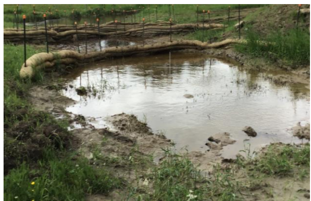
Sediment fences, sandbags, straw wattles and berms observed to control sediment.
