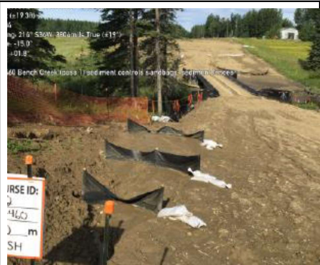
Bench Creek temporary travel way during construction.
