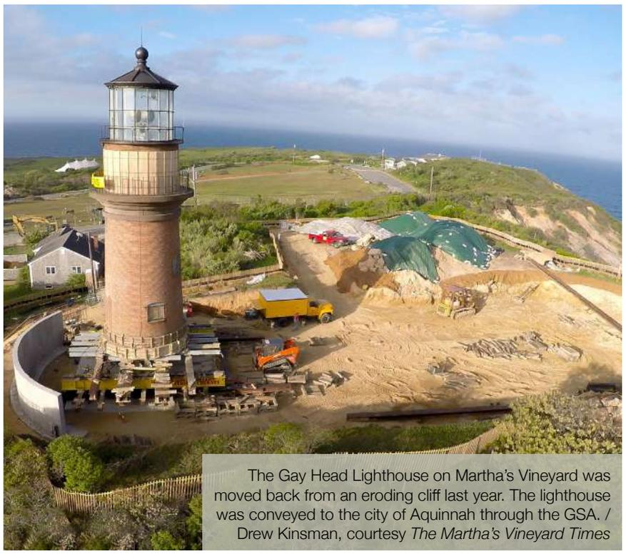
The Gay Head Lighthouse on Martha's Vineyard was moved back from an eroding cliff last year. The lighthouse was conveyed to the city of Aquinnah through the GSA. / Drew Kinsman, courtesy *The Martha's Vineyard Times*
