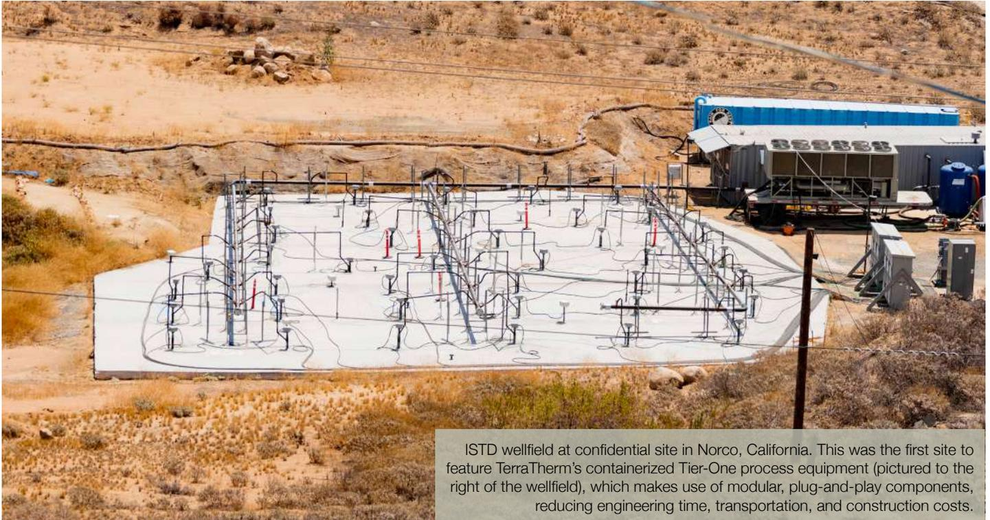
ISTD wellfield at confidential site in Norco, California. This was the first site to feature TerraTherm's containerized Tier-One process equipment (pictured to the right of the wellfield), which makes use of modular, plug-and-play components, reducing engineering time, transportation, and construction costs.
