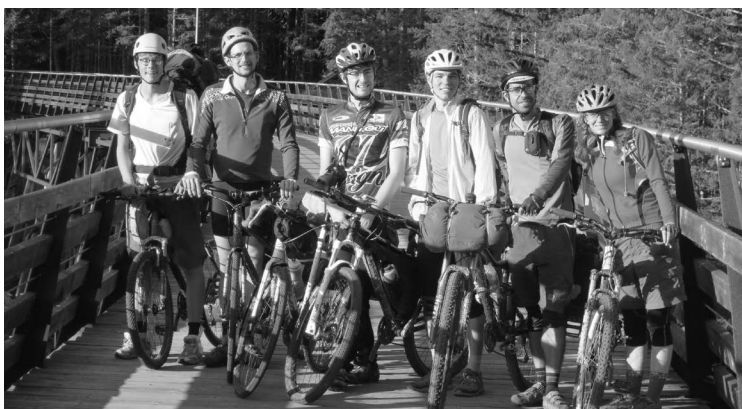
The team on the Kinsol Trestle near Shawnigan Lake.
