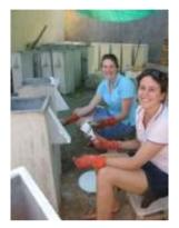
Volunteers helped minimise this problem by assisting in the construction and provision of bio-sand water filters. They are a low cost way to provide potable water from any water source to impoverished areas. The volunteer work also included working
