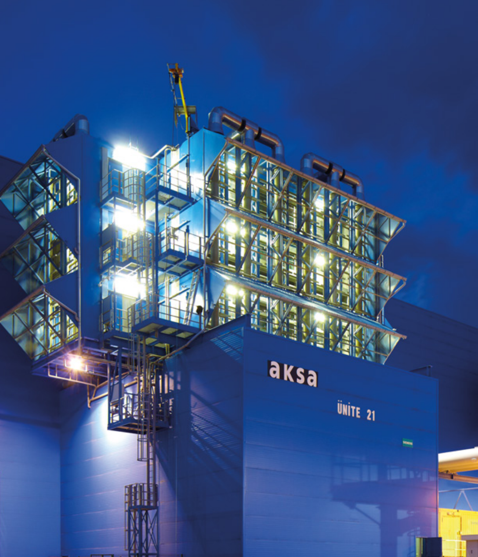
Ali Metin Kazancı Antalya Natural Gas Combined Cycle Power Plant
