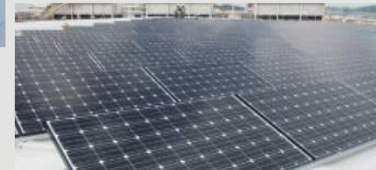
Photovoltaic facility at Ochang Plant
