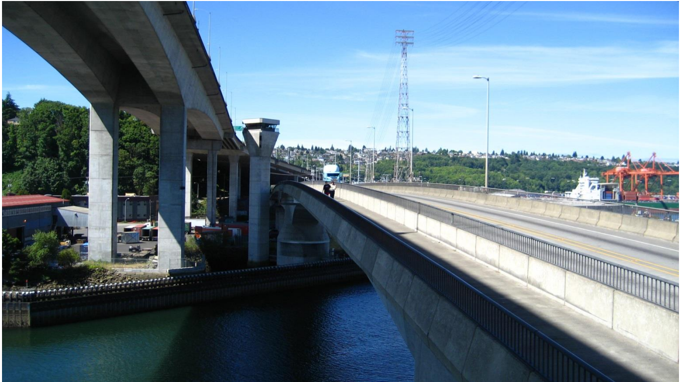
Figure 8: Lower Spokane St Swing Bridge
