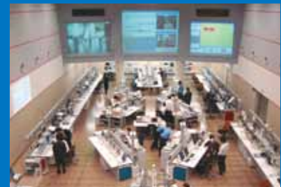
Integrated Control Room of Tatebayashi System Center
